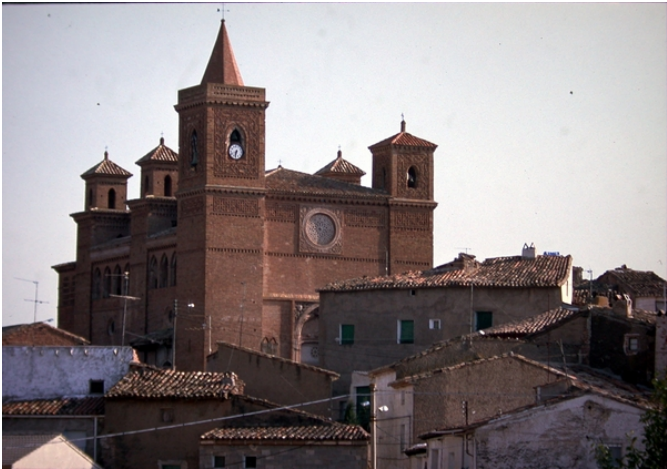
Vista exterior general
