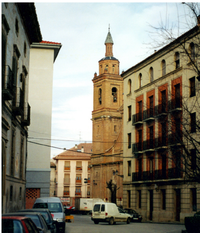
Vista parcial fachada principal
